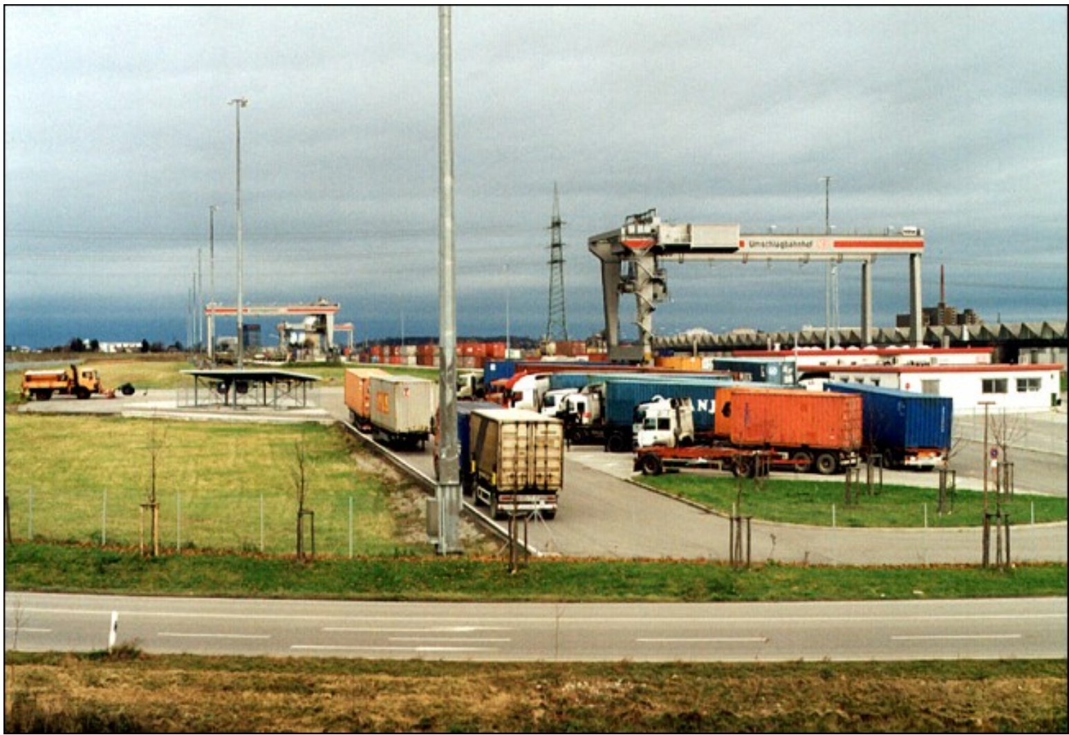
Fig. 4/2: Container terminal Kornwestheim
